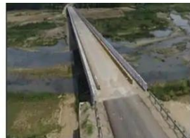
TARNAH-II BRIDGE (300 m)
