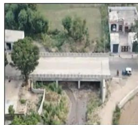
PANYALI BRIDGE (31 m)
