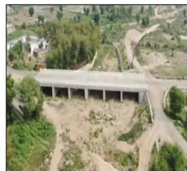
PAHADIWALA BRIDGE (61 m)
