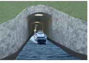
The Norwegian Coastal Administration has received the green signal to start working on the construction of **world's first tunnel, being built exclusively for ships.**The tunnel is dubbed as **"Stad Ship Tunnel"** and would be built under the mountainous Stadhavet peninsula in northwestern NorwayThe 1.7 km tunnel will be able to handle ships of up to 16,000 tonnes and give ships a safer passage through the
